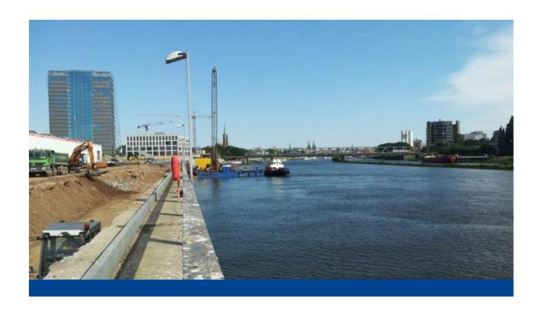
Construction of a new Quay wall in front of an existing structure in the vicinity of "Weserbahnhof 1" in the City of Bremen with a length of 356 m, consisting of a combined steel sheet pile wall, anchored by inclined micropiles including equipment, super-structure as well as flood protection wall, reinforced concrete wall and steel wall. The project included these main components:
