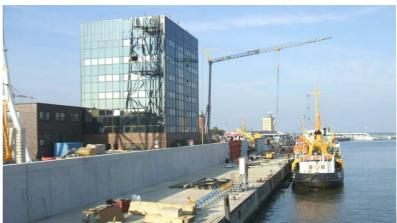
The existing dike line will be shortened and at the same time adapted to a higher level of protection. On land, this will be achieved by concrete structures, wave sheet piling and the installation of storm surge gates.
