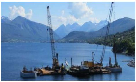
The work on the foundations in the North sea fjord, which is up to 40-meters deep, presented a special challenge to Marine. The 13 bridge piers rest on foundations that consist of specific configurations of tubular steel piles filled with concrete and measure 1.22 meters in diameter. In total a full 9.000 meters of steel tubing were needed for the piles.
