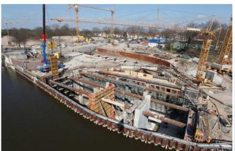
Construction of a hydropower plant as a bypass structure next to the Weser weir in Bremen.
