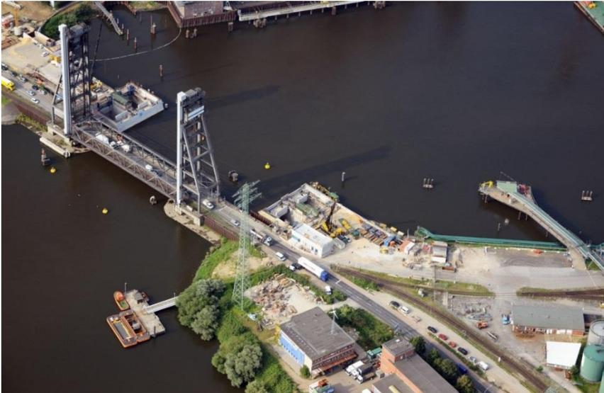
The port of Hamburg gets one of Europe's largest bascule bridge, accommodating both, railway and road traffic. The bridge spans a branch of the River Elbe and is an important link inside the port. It replaces an existing lift bridge following 75 years of service.
