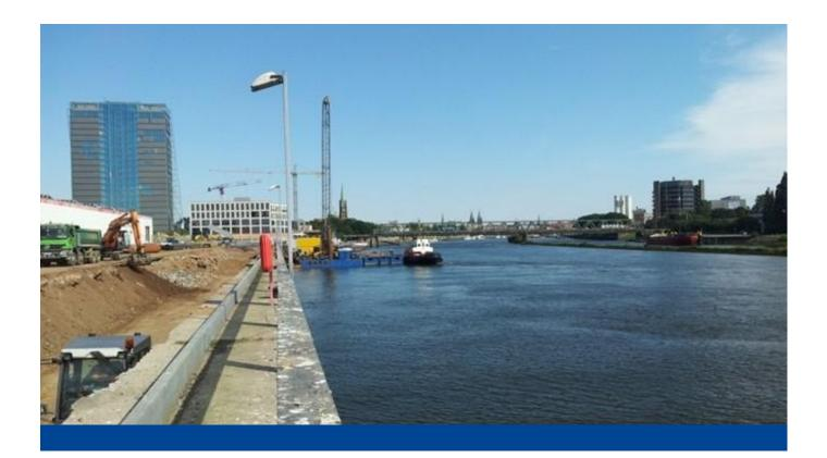
Construction of a new Quay wall in front of an existing structure in the vicinity of "Weserbahnhof 1" in the City of Bremen with a length of 356 m, consisting of a combined steel sheet pile wall, anchored by inclined micropiles including equipment, super-structure as well as flood protection wall, reinforced concrete wall and steel wall. The project included these main components:
